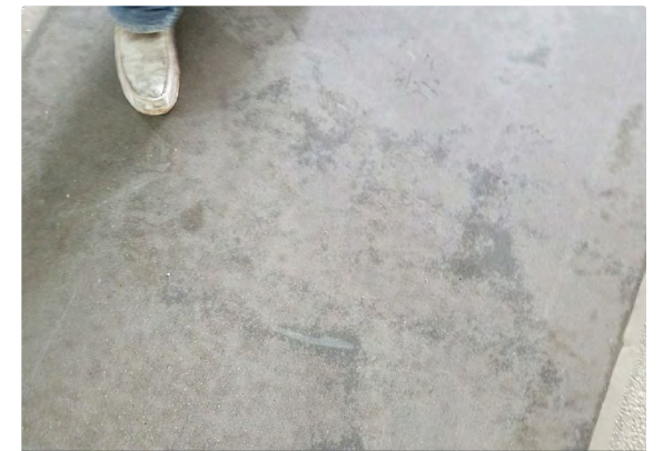
Concrete floors typically have an uneven appearance.
